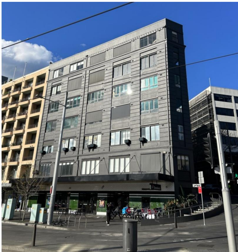
Figure 4 – View of Chalmers Street Frontage of Existing Building – 17 Randle Street (Source: City of Sydney)
